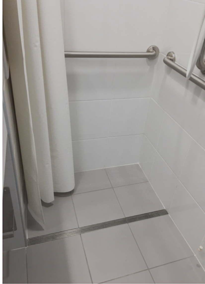
QuickDrain ProLine Drain System installation at a major Cleveland, Ohio hospital
